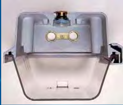
Bolted through suspension points & fully compressed gasket
